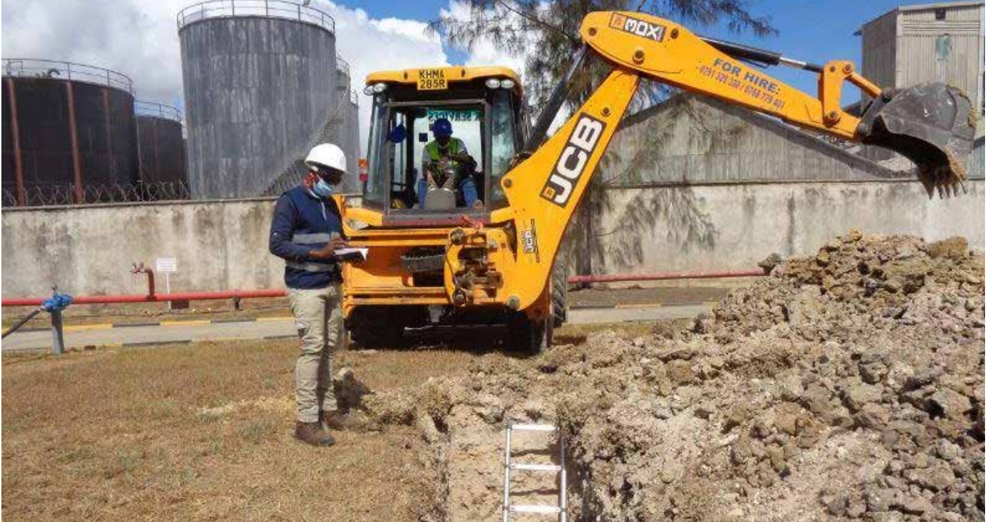
Excavation of trial pit - Mombasa county
