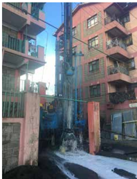
Drilling in progress at umoja borehole for client Mr. Joseph Ngaruiya Mbua,
