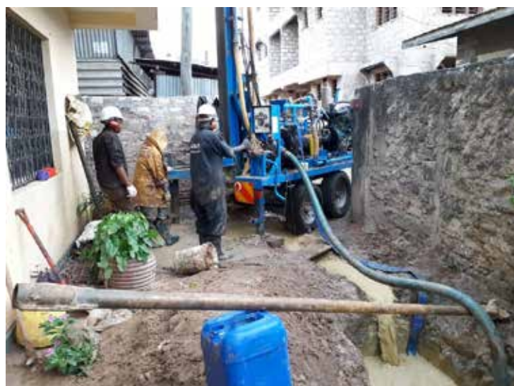
Mud drilling in progress within Mikindani area
