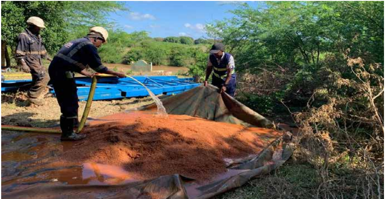
Cleaning gravel pack before insertion in the borehole
