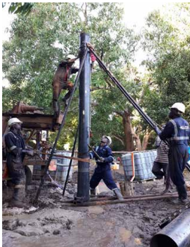
Installation of 10" Casings and screens
