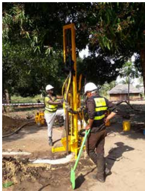
Mud drilling in progress using the potable PAT 301 Rig in Majoreni area of Kwale County
